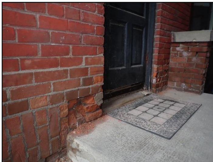
Some deteriorated brick noted
