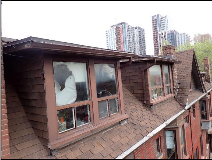
Shingles at or near end of life
