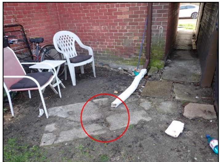
Maintain discharge well away from foundation
