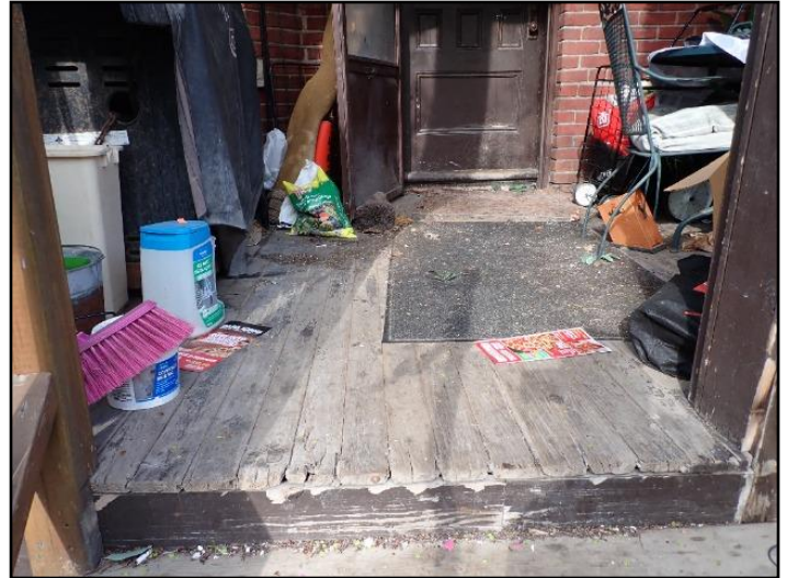
Porch flooring is weathered/worn
