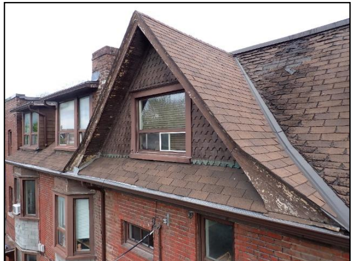
Shingles are in generally poor condition
