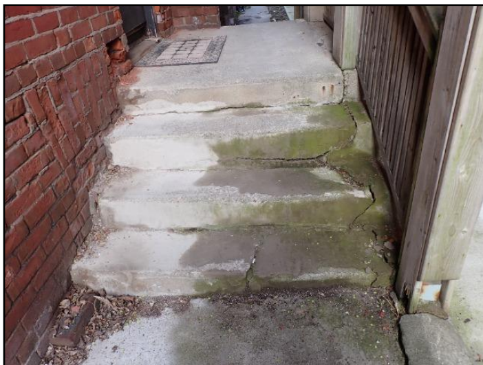
Steps are cracked/settled
