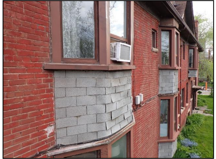
Loose, worn shingle siding
