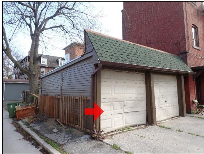
Damaged garage door
