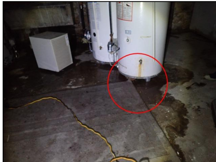
Leaking water heater
