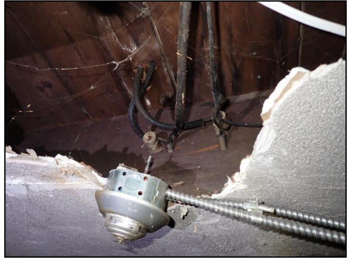
Knob-and-tube wiring
