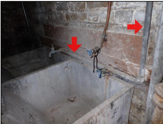
Galvanized steel piping
