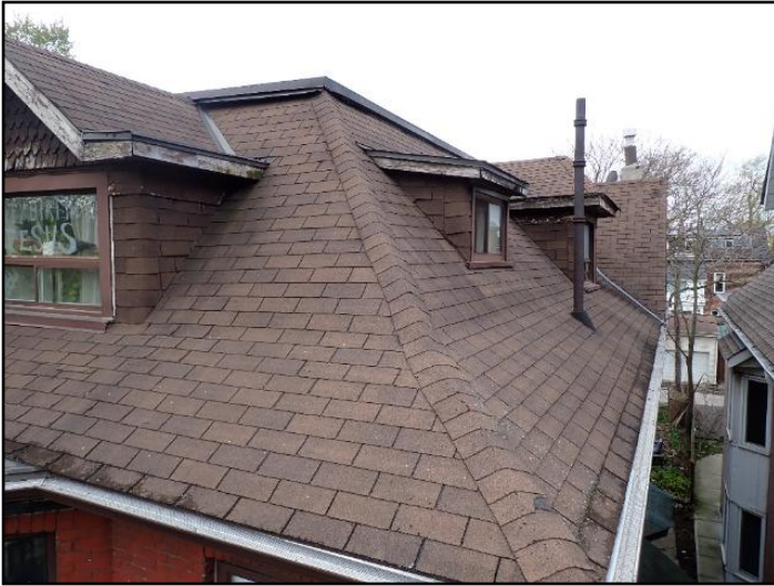
Shingles are in generally poor condition
