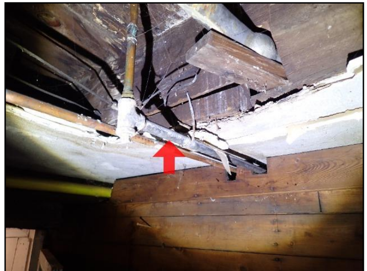
Galvanized steel piping
