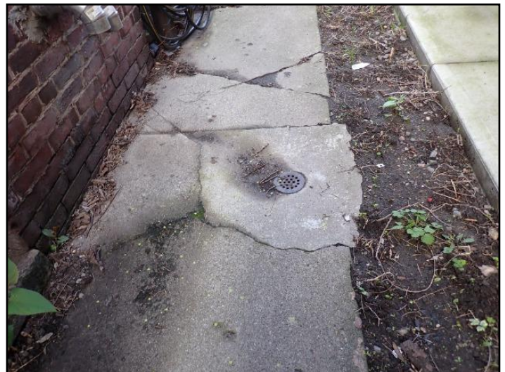
Sidewalk is cracked
