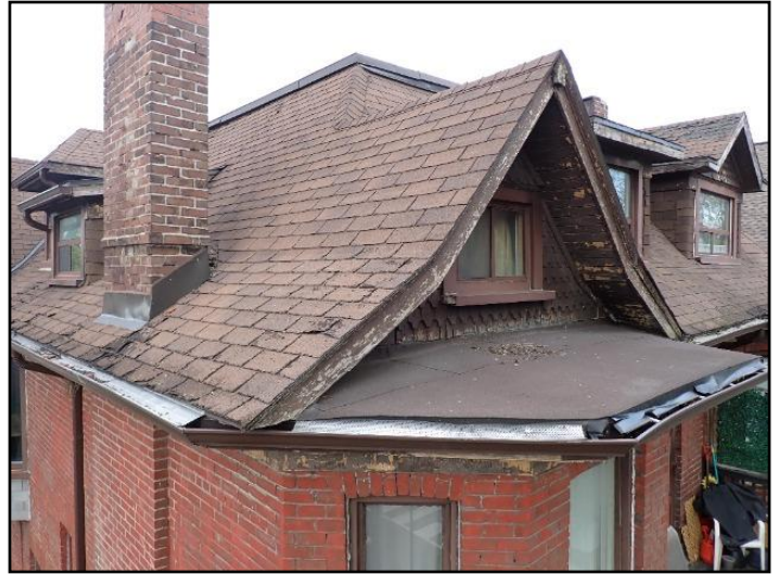
Shingles at or near end of life
