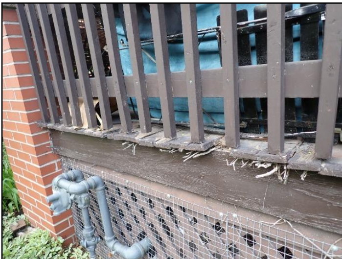
Porch flooring is weathered/worn
