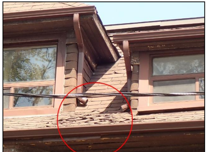
Damaged shingles
