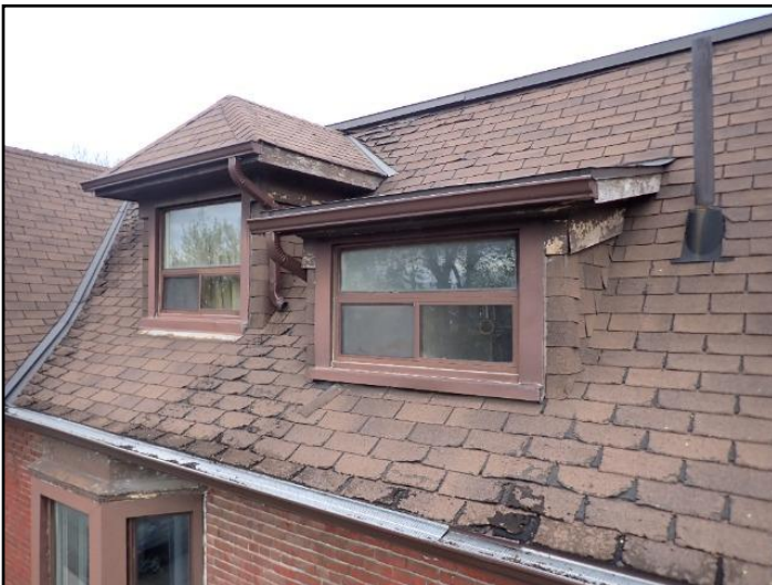
Shingles are in generally poor condition
