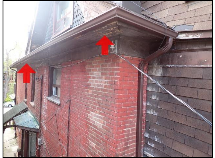
Soffit/fascia could be capped to lower maint.
