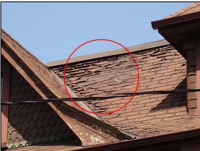
Damaged shingles
