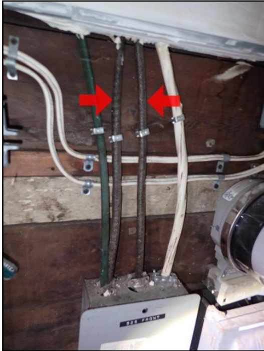
Knob-and-tube wiring
