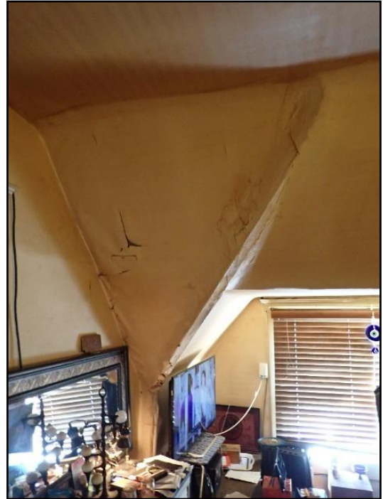
Tenant reported stains from roof leak
