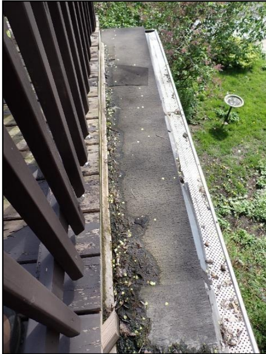
Cracked surface of flat roof under deck
