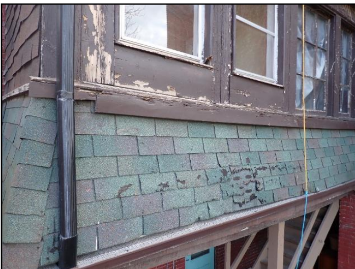
Worn shingle siding
